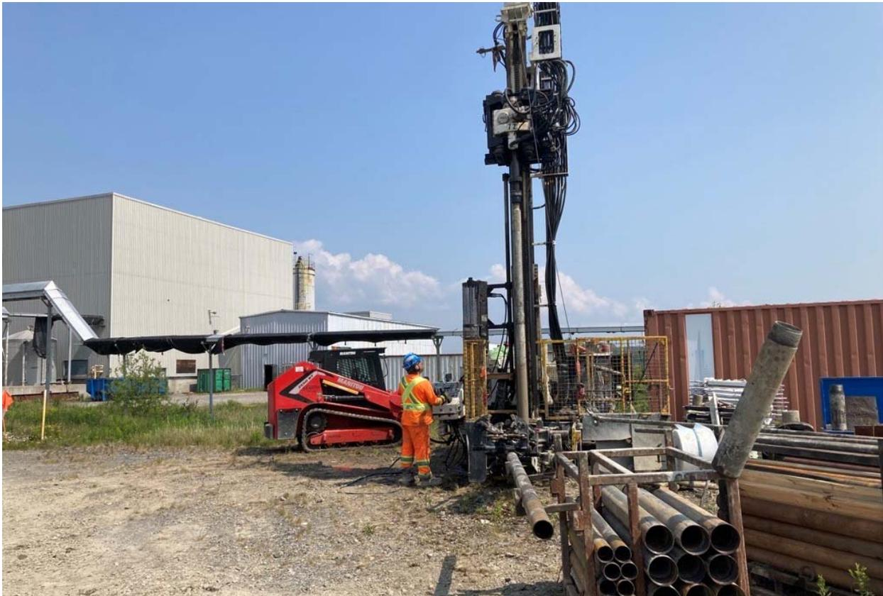
**Figure 1. Boart Longyear drillers collect geotechnical data for design of the solvent extraction plant**
