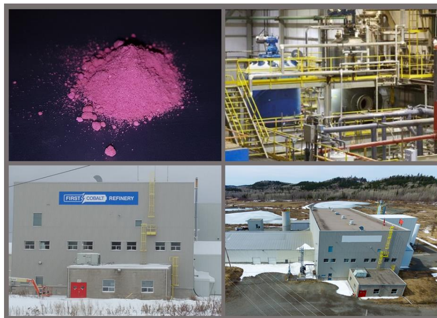
Image 1. First Cobalt Refinery exterior, interior and cobalt sulfate material
