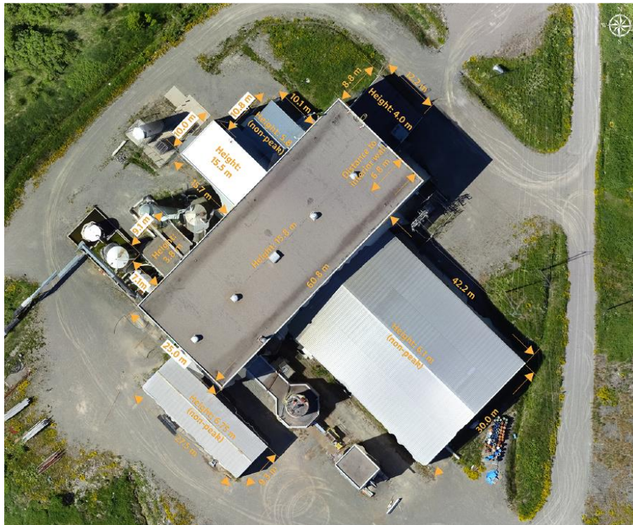
Figure 1 – First Cobalt Refinery Aerial View
