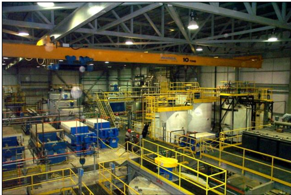
Figure 2 - Interior of Yukon refinery
